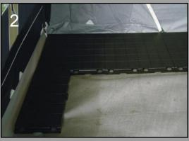
Lay the IKAFLOOR plastic flooring, ensuring that the rows are staggered. Begin in the left-hand corner and lay floor tiles along the length of the caravan. Start every second row with a half tile.
